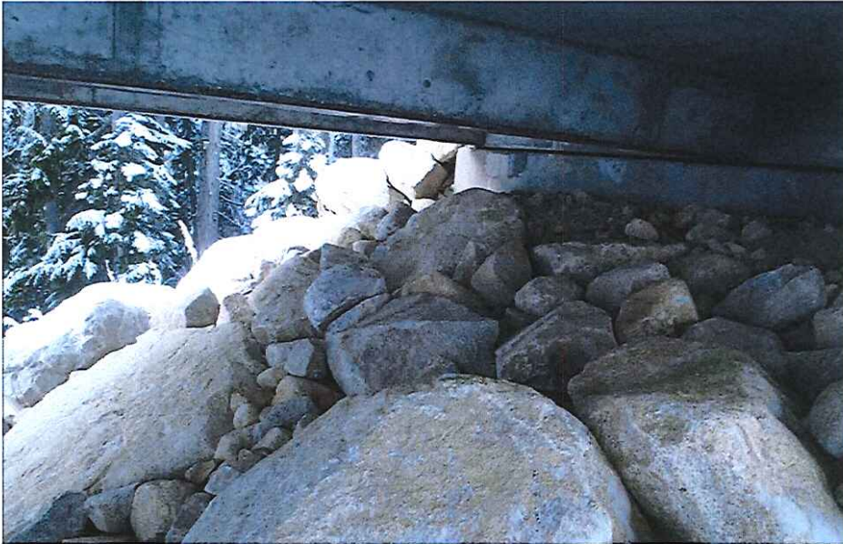
CK2361 Right abutment
