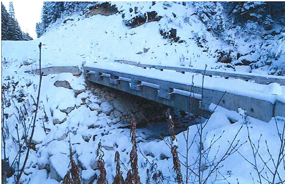
CK2361 from downstream
