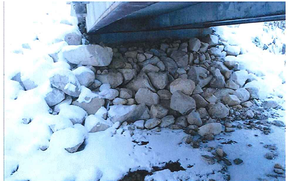
CK2361 Left abutment
